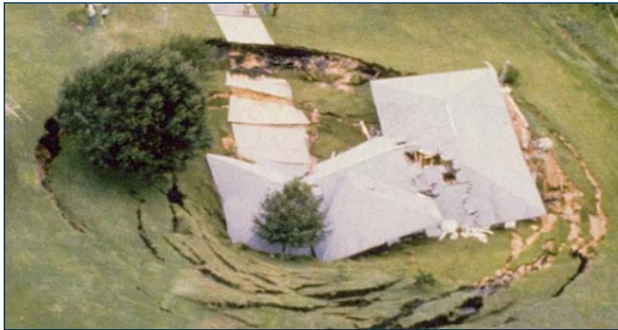
No Question: Sinkhole Damage
